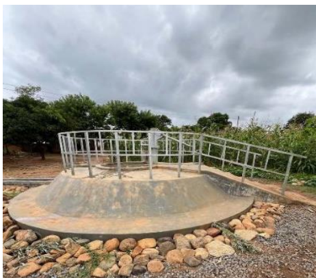
Image 1: Re-designed climate-resilient handpump
